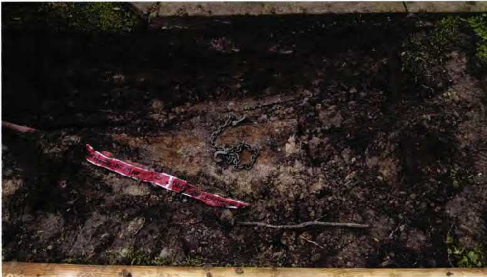
Picture 2: UST 252Beech excavation.
