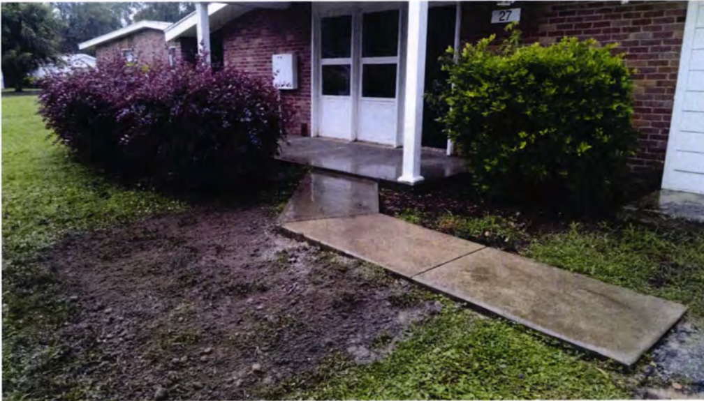
Picture 3: Site after completion of work.
